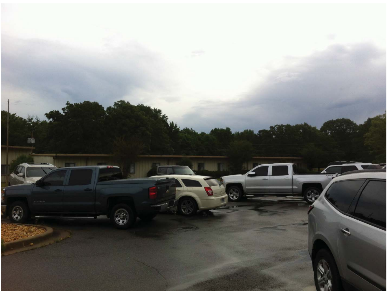
Building 798, Side View, East Side
