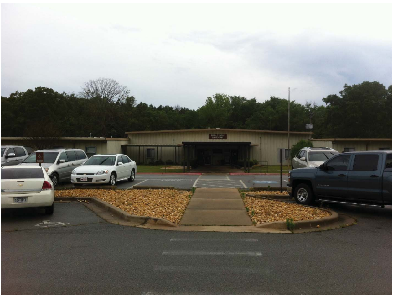
Building 798, Front of Building
