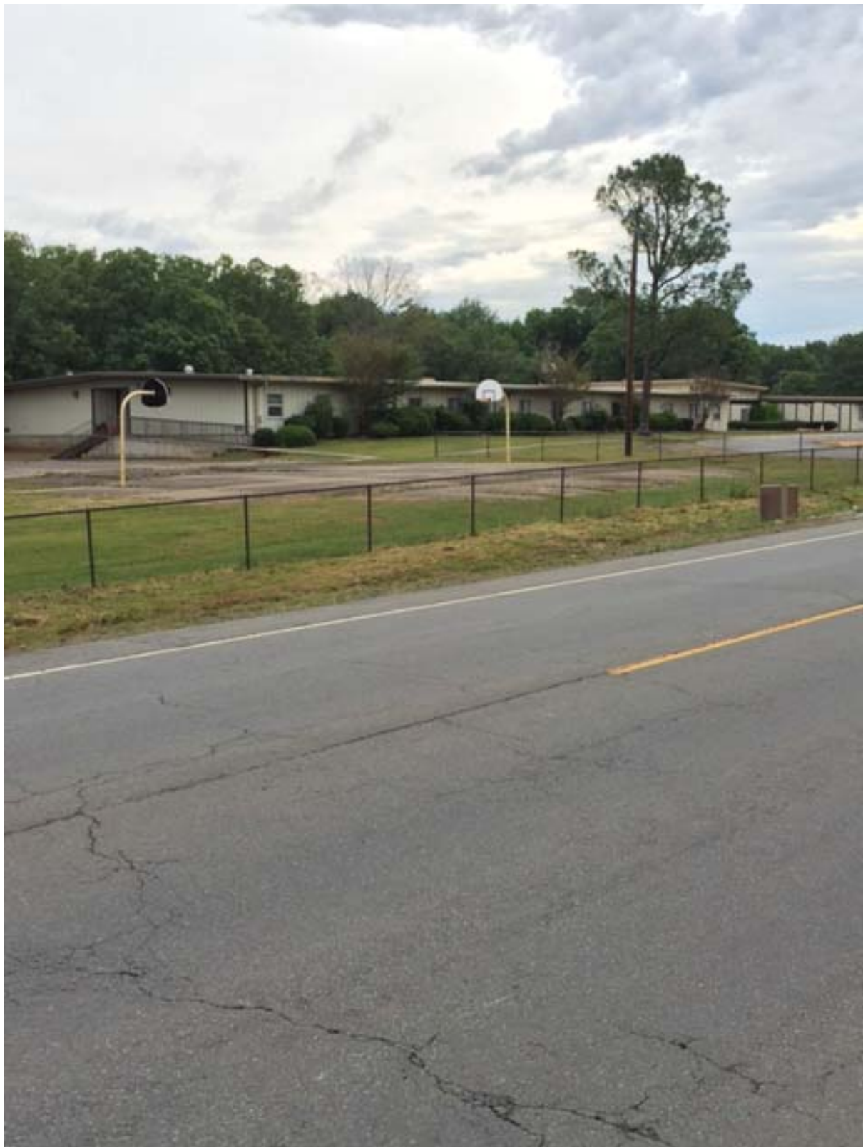
Building 798, North Side
